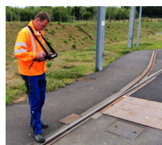
Visual inspection of switch
