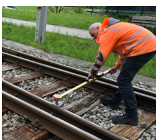
Taking measurements on a switch
