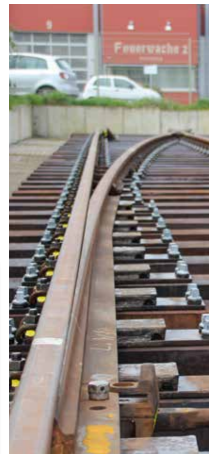
Turnout installation in Dortmund
